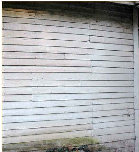
Photo #26 House, View #26, West Elevation, Detail of Siding, Camera Facing East; note the joint lines in the siding
