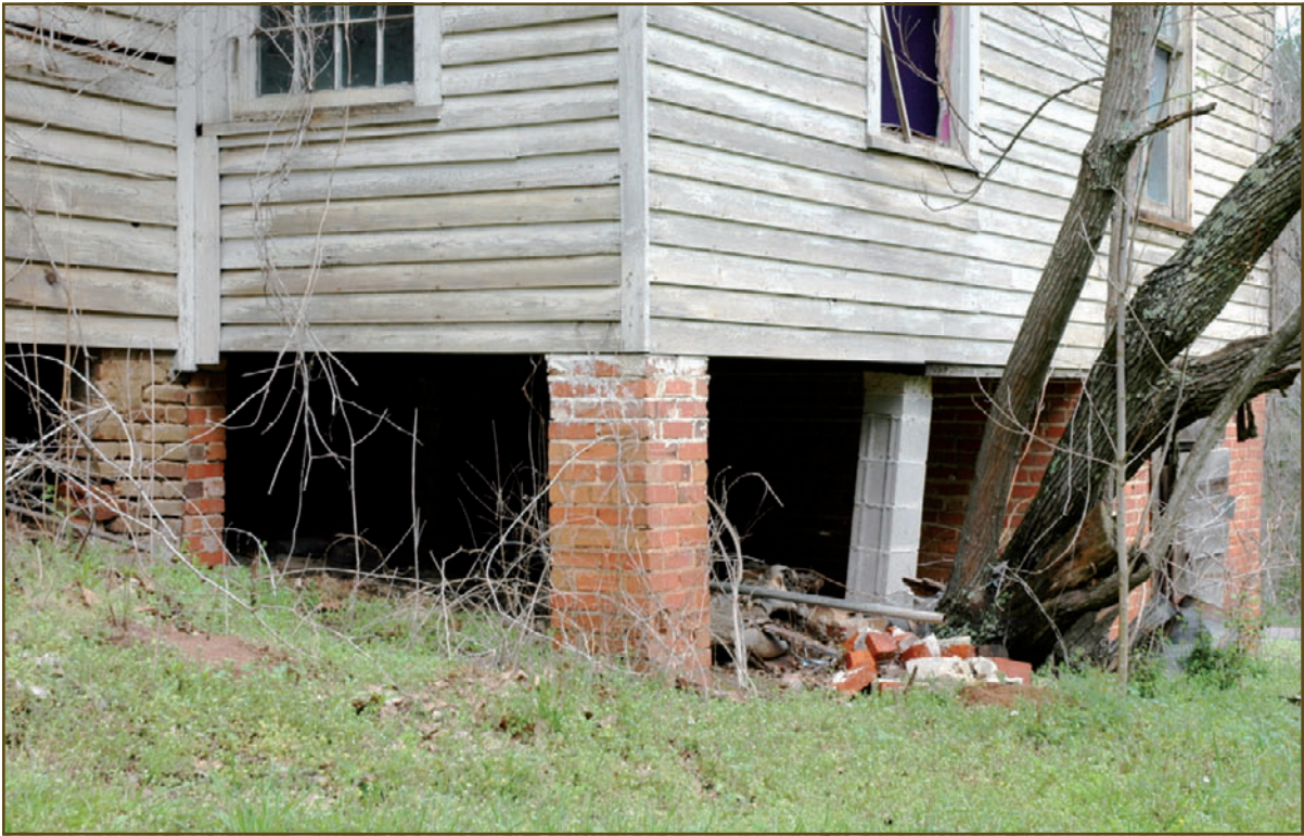
Photo #27 House, View #27, Detail of Brick Piers, Southwest Corner, Camera Facing Northeast
