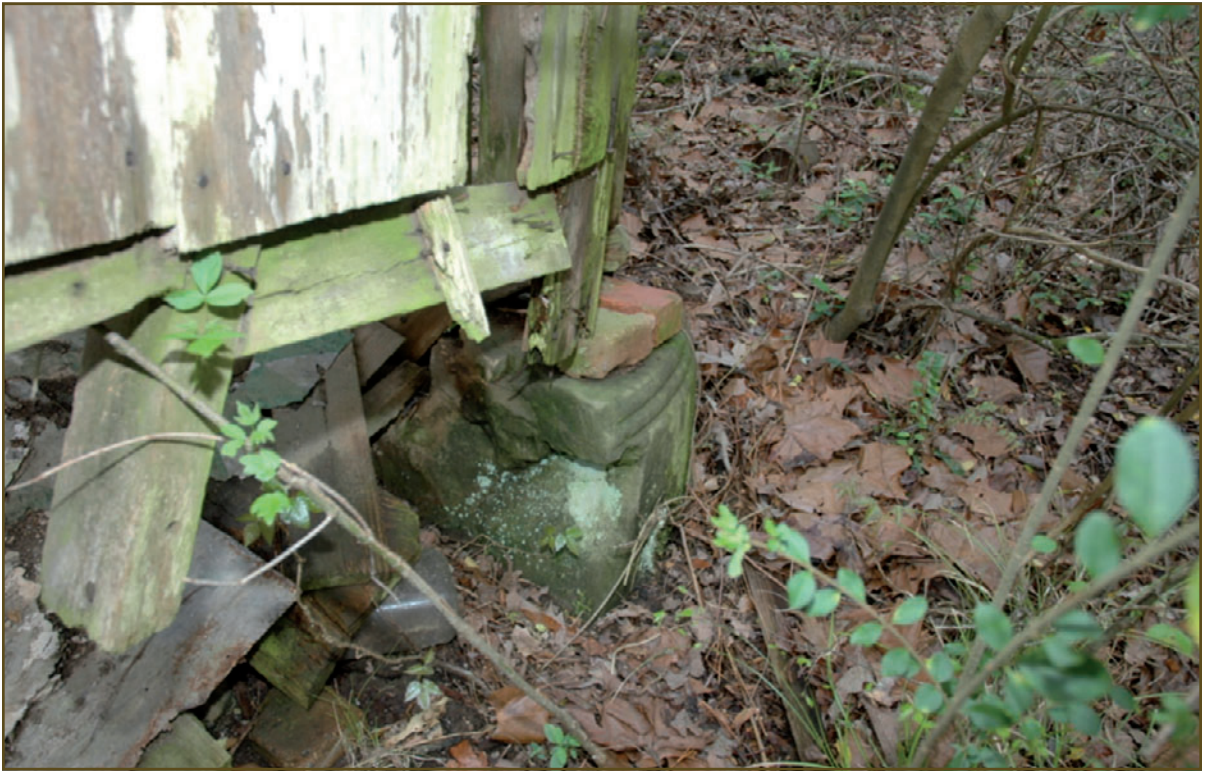
Photo #64. Shed, View #7, Detail of Stone Pier (Possible remnant of an old mill stone?)
