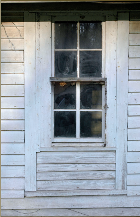
Photo #24 House, View #24, West Elevation, Detail of Window at Rear Extension, Camera Facing West; note the former entrance opening with infill
