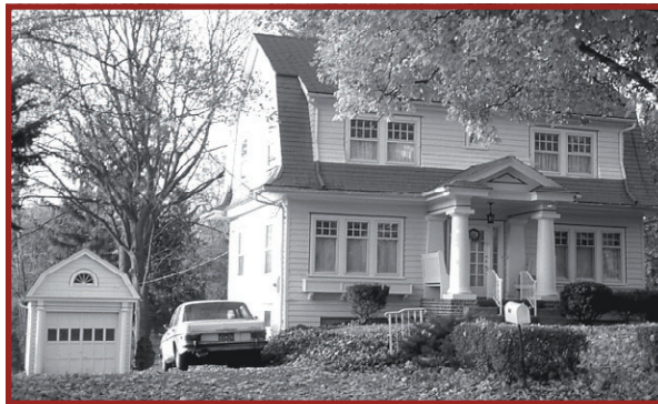
8.2 Note how outbuildings can be an important element of the overall character of a property in the district.
